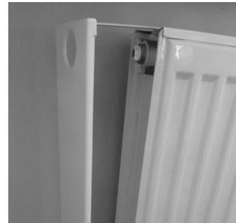
2. After the side cover has been taken off, lead the current-carrying conductor and the power supply conductor of the fan modules through the opening designed for the radiator's upper connector, and fix the controller's case with adhesive elements (to be found at the back of the controller's case).
